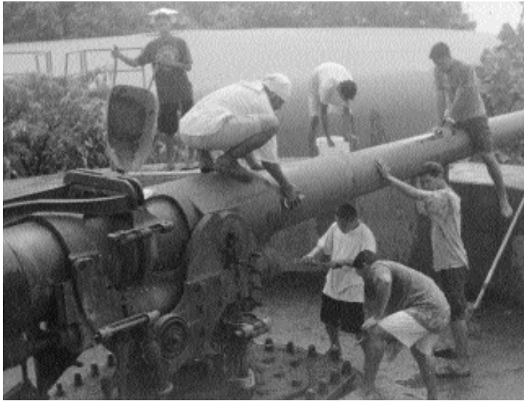
Boy Scouts clean the concrete gun enclosure and remove rust from the lower Blunts Point Gun using sandpaper and wire brushes. December 1999. Photo by Analosa Vele.
